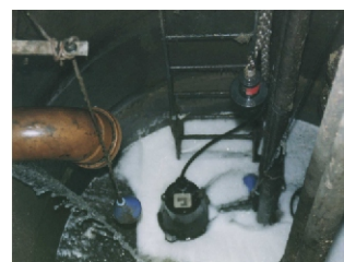
Sewers and drains which are inaccessible for foam detection
