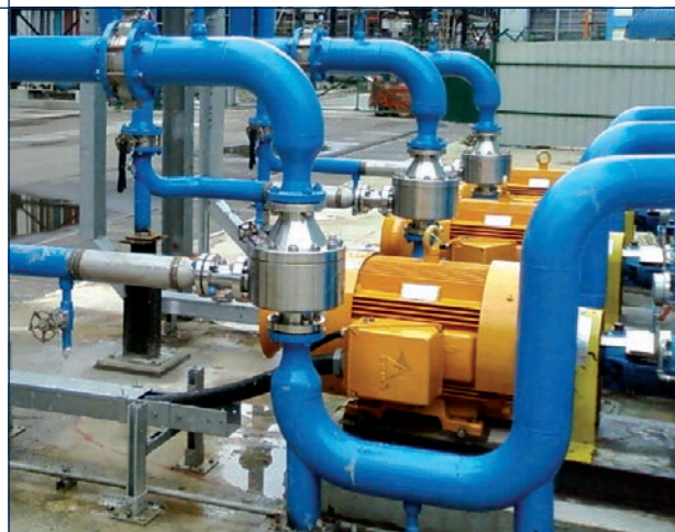
SureFlo™ in a boiler feedwater application
