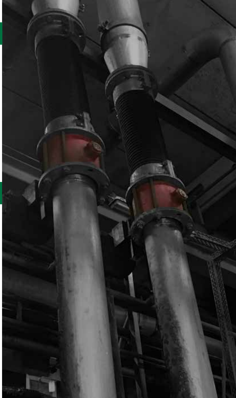
Ramén Ball Sector Valve KSG installed in a mining facility
